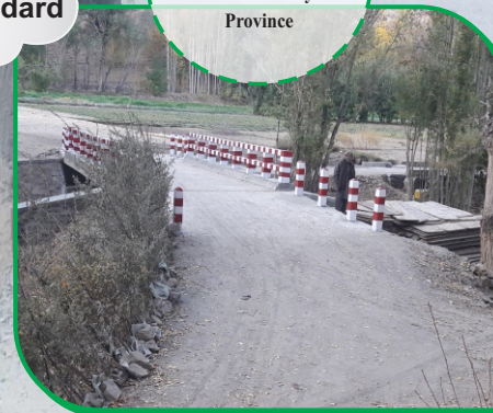
Construction of 10 Rm RCC bridge in Waras District of Bamyan Province
