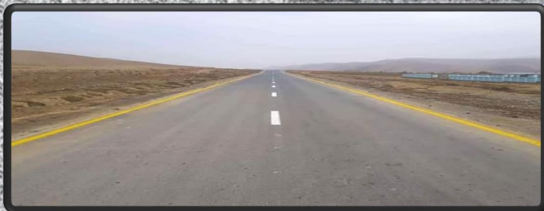
Construction of 10.2 km of Road in Bangi district of Takhar Province by NRAP.MoPW
