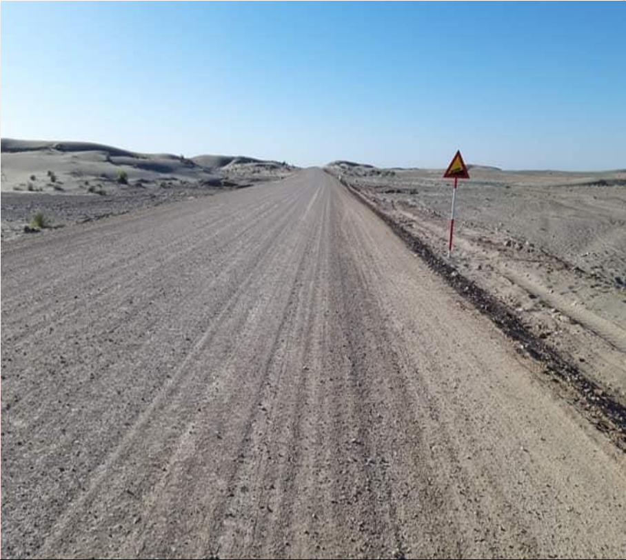
Construction of 9.140 km road in Qarqin ditrit of Jawzjan Province by NRAP.MoPW
