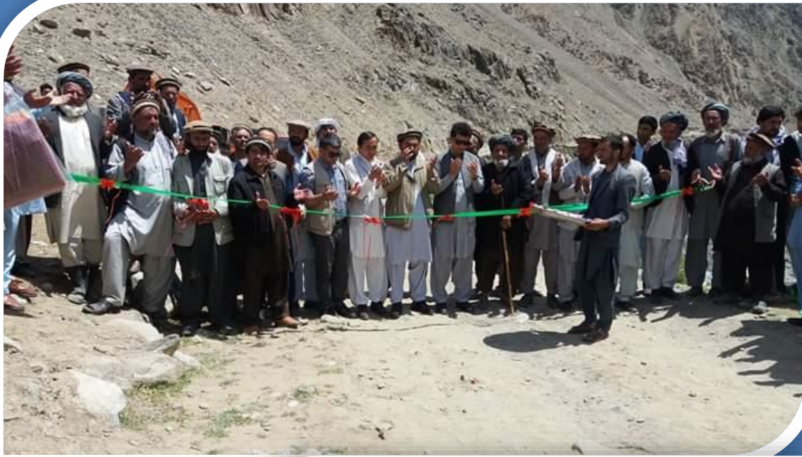
Construction work inauguration of 20 KM gravel surface road in Warsaj district of Takhar Province by NRAP.MRRD
