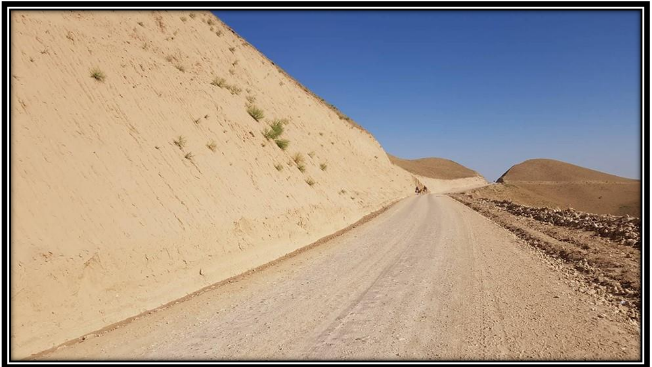
Construction of 8 Km Road in Pashtoonkot district, Faryab Province by NRAP.MoPW
