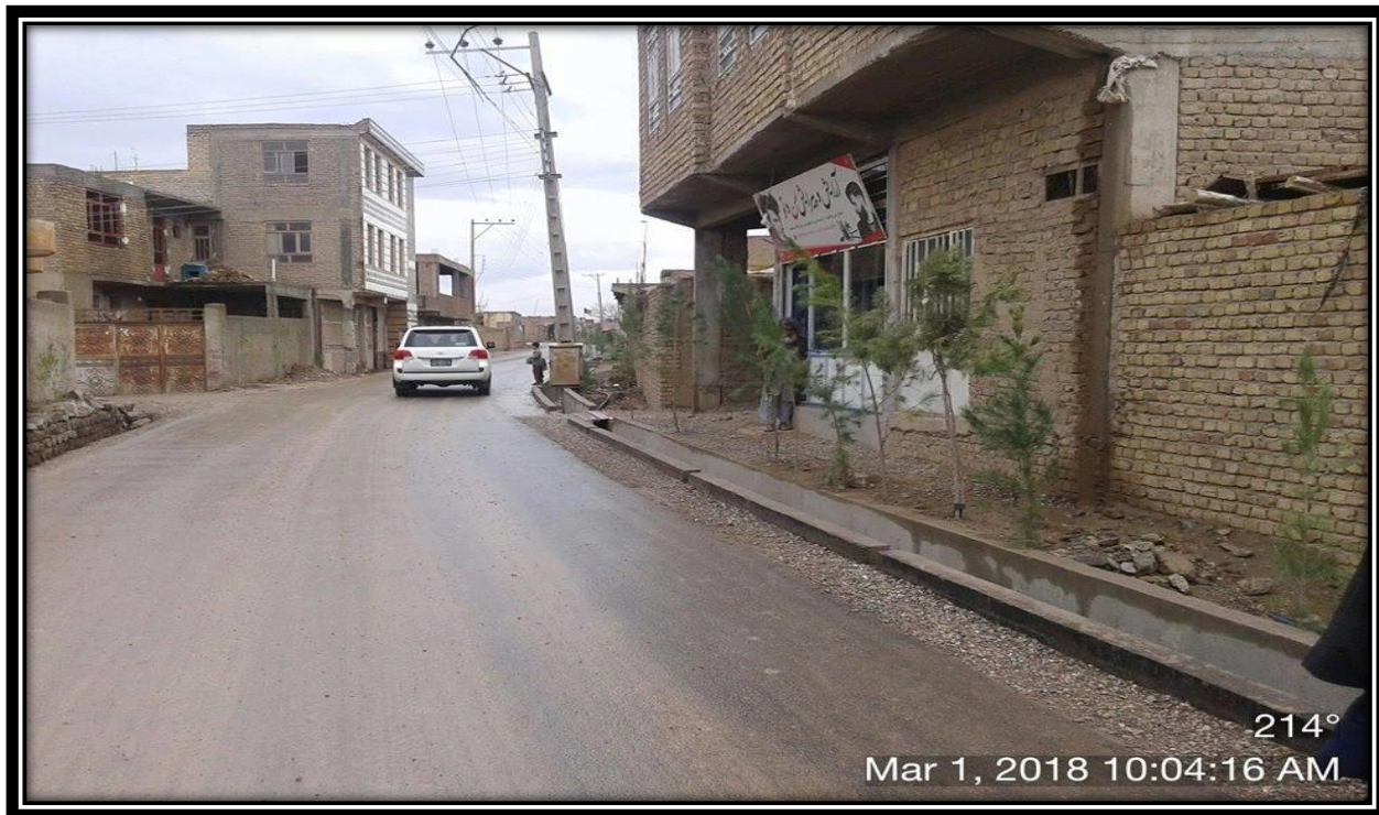
Construction of 1.77 Km Road in Injil district, Hirat Province by NRAP.MRRD
