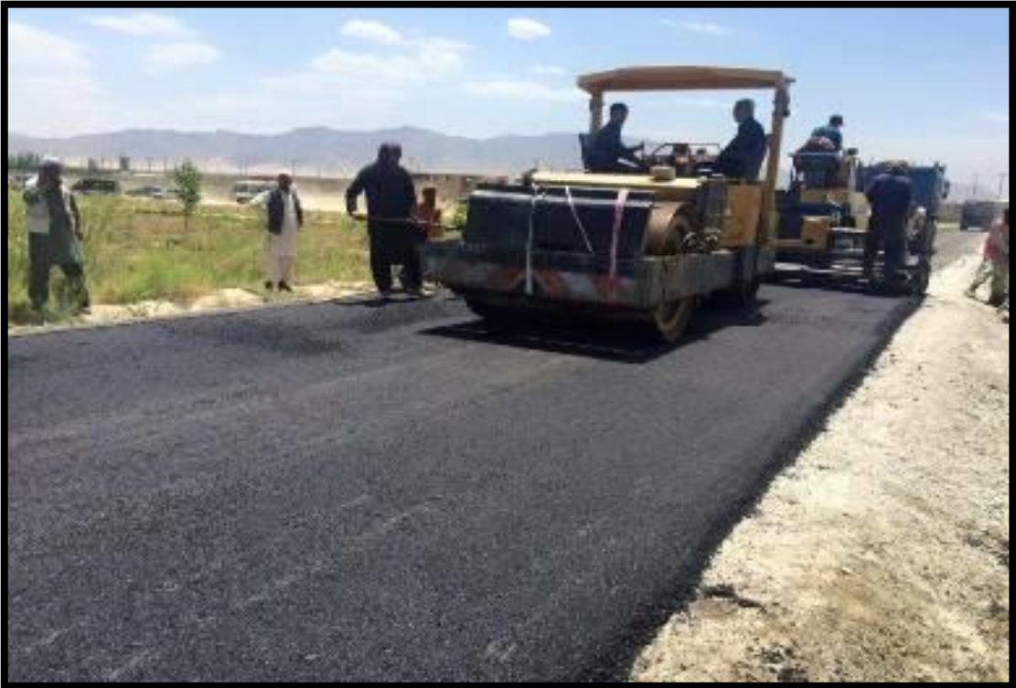
5.2 Km Road in Bagram District of Parwan Province
